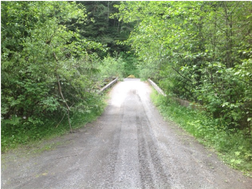
Right Bank Abutment when facing downstream
