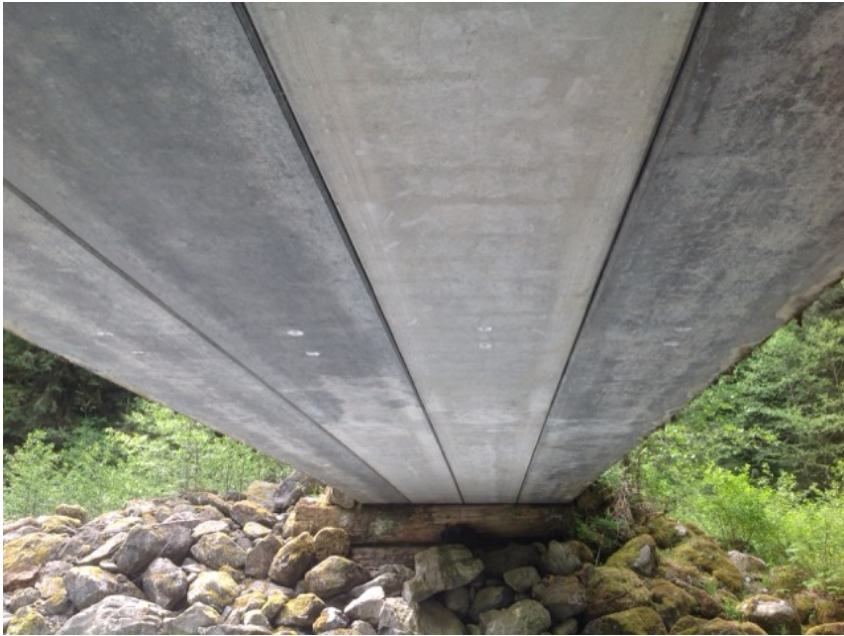
superstructure - 4 concrete slabs
