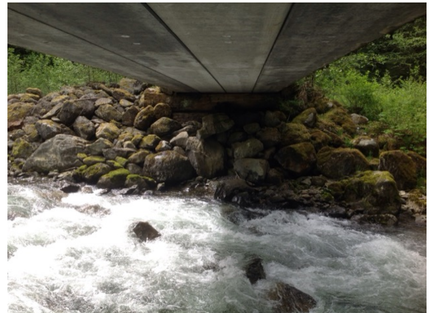
Left Bank Abutment when facing downstream
