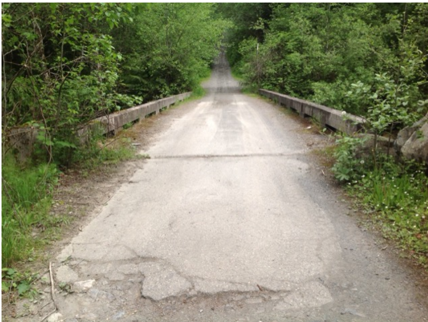
Approach from Left Bank when facing downstream - paved approach
