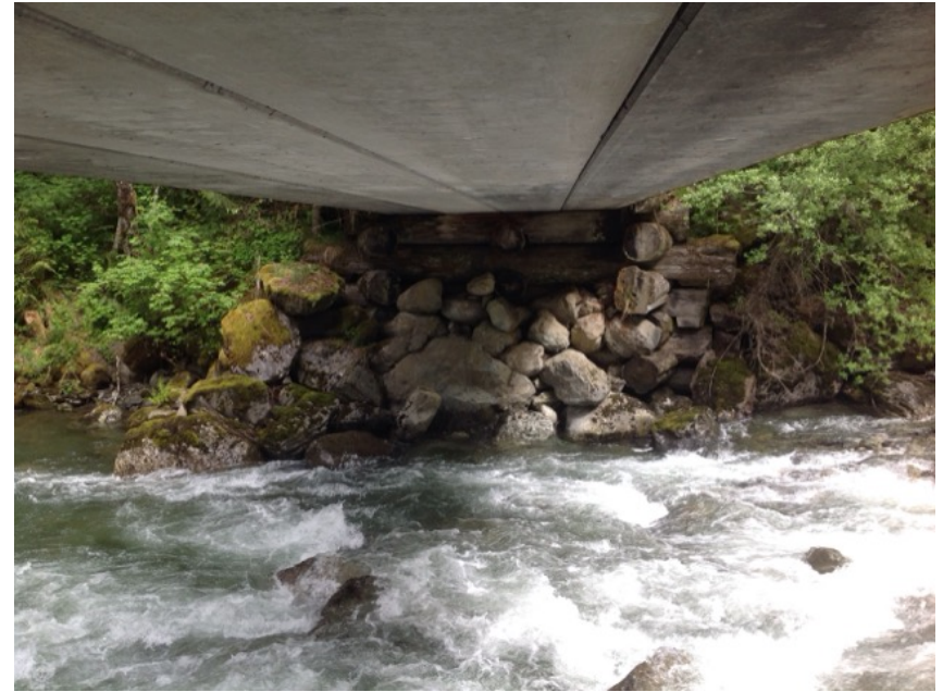
Right Bank Abutment when facing downstream
